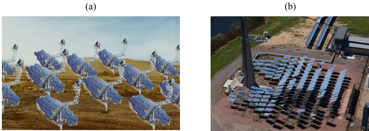
7 Figure 3.10: (a) Rendering of aggregated dish/Stirling units, and (b) a solar tower for powering a 8 Brayton cycle microturbine (courtesy CSIRO).
