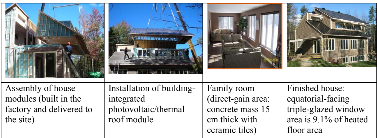
19 Figure 3.4: Photos from the EcoTerra™ demonstration solar house assembly and the final 20 completed house. [TSU: source missing]
