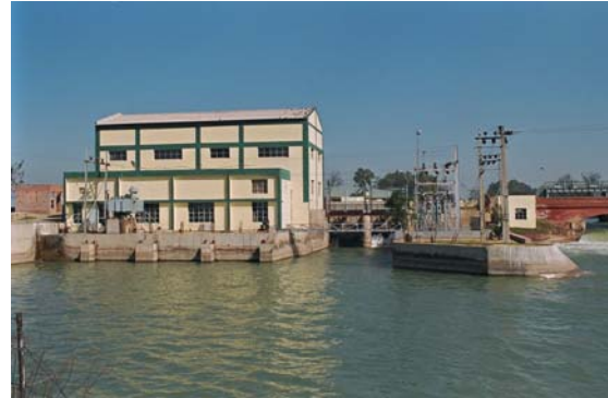
7 8 Figure 5.9: Typical arrangement of instream technology hydropower projects. (Narangawal,, India)
